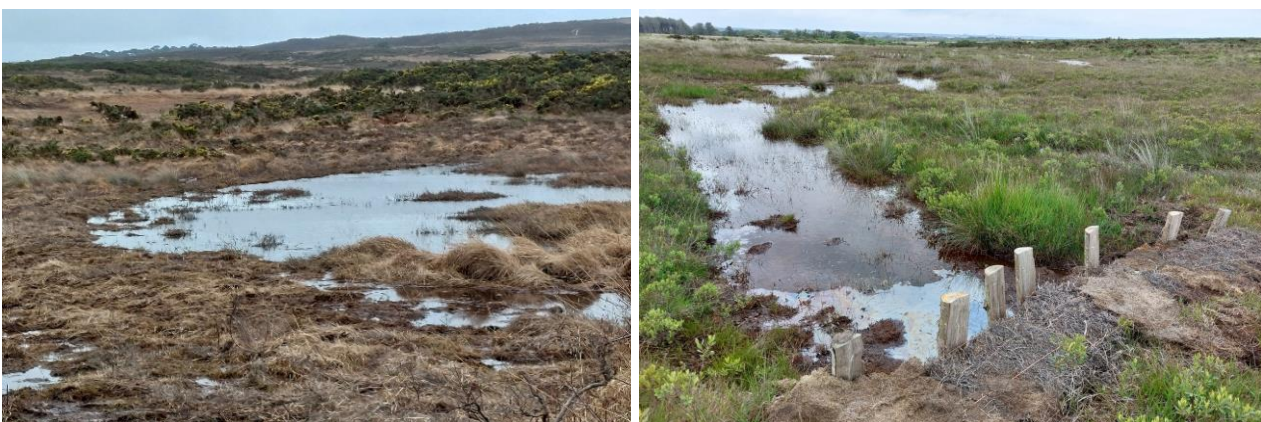
Peat bunds and heather bale dams were created to slow the flow of water through the valley mire (Site B-recently restored site).
