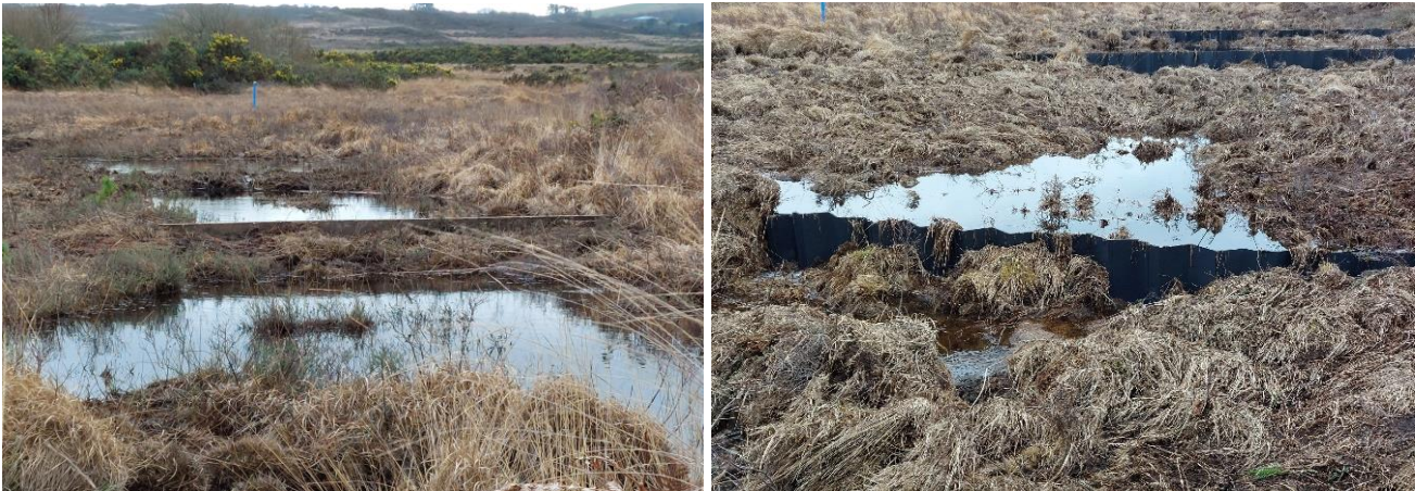
Photos showing the plastic and timber dams used in the restoration project (Site B-recently restored site) to block the incised channels draining the mire. Taken post-restoration on the 20 th February 2024.
